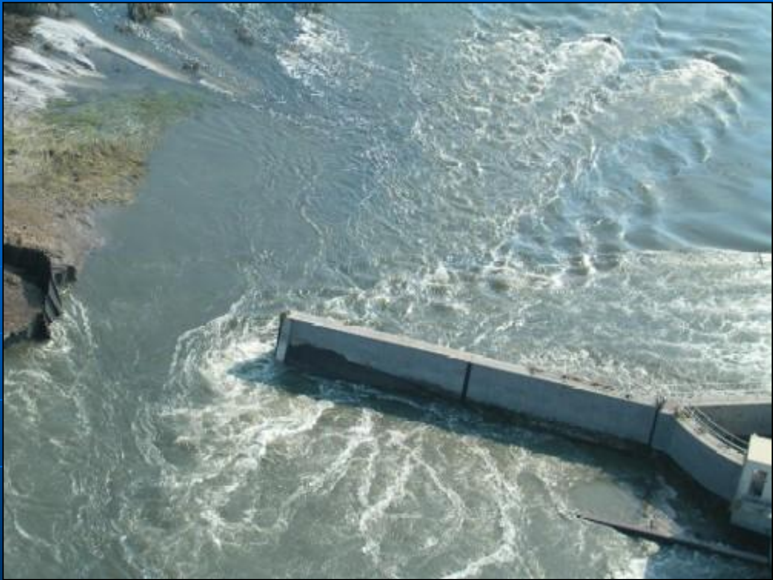
East Side IHNC North Breach, near Florida Ave. bridge and pumping station, during inflow. Note narrow chasm defined by this failure and dramatic flexure of the sheetpiles.
